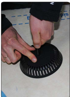
Overdelen presses ned mod undertaget.
